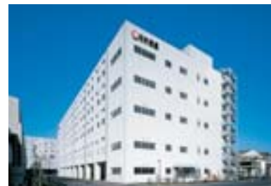
A distribution facility
