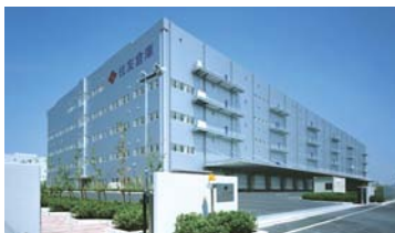
A distribution facility
