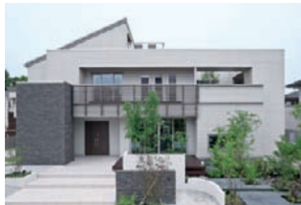
The SMAxEco HOUSE at our Yagoto display site, Aichi Pref.
