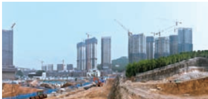
The Yihe Xinghai project under construction in Dalian
