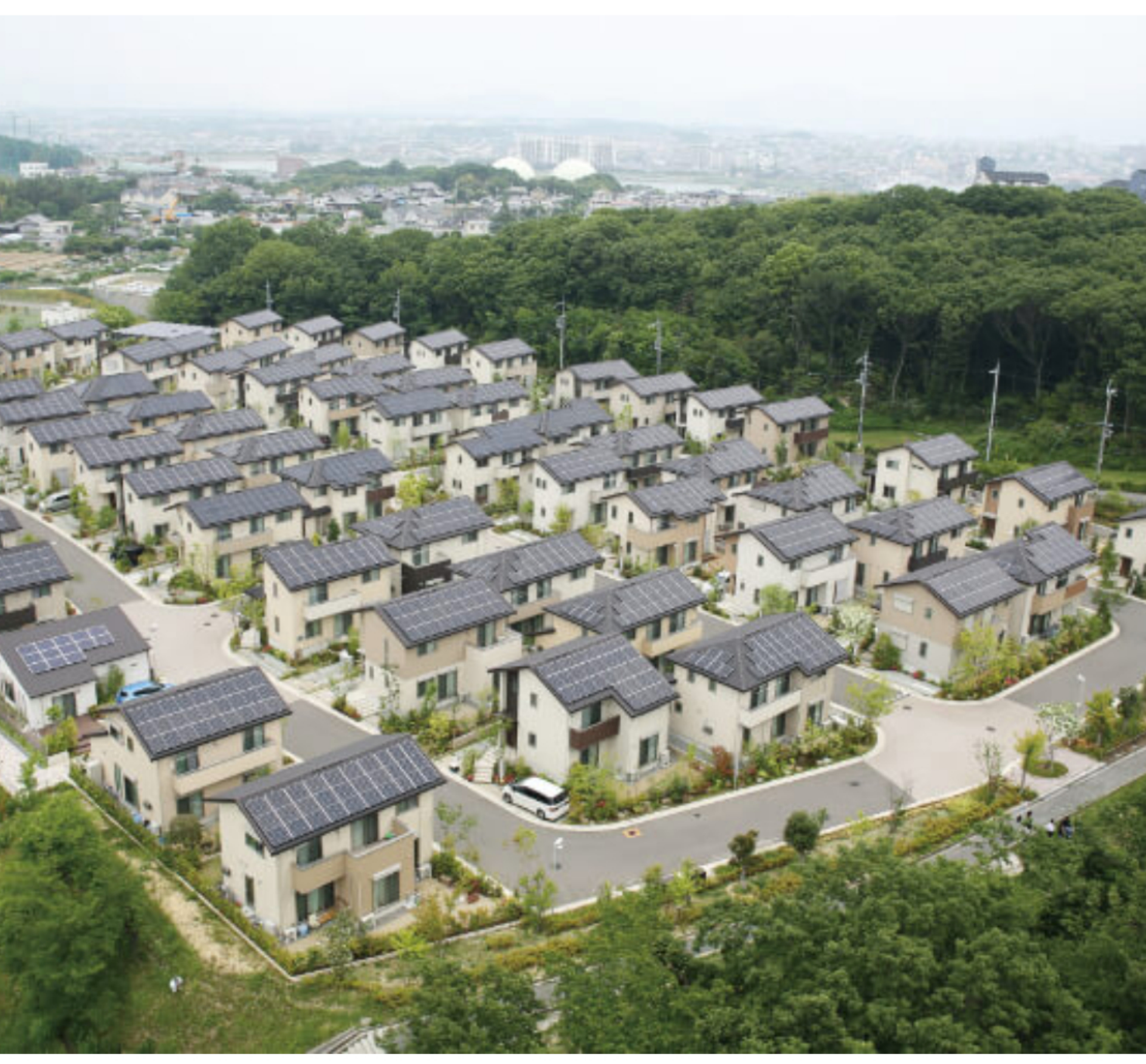
A net-zero energy town (ZET), where all homes are equipped with solar photovoltaic power units with lithium ion storage batteries and where a state-of-the-art energy management system is used to ensure net-zero energy consumption across the entire town. (Photo: SMA Eco Town Harumidai)
