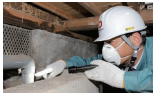
Underfloor space inspection
