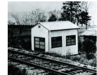
Following a major typhoon that destroyed and damaged large numbers of wooden structures, Nobuo Ishibashi noticed how both bamboo and rice, which have hollow stems, were able to bend flexibly and gracefully despite the fury of the wind, without breaking. This gave him the idea of a steel-pipe structure, and the Pipe House pioneered the subsequent industrialization of construction in Japan, by which the country's construction industry was revolutionized.
