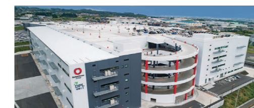
The largest earthquake-resistant multi-tenant logistics facility in Shizuoka Prefecture with a nursery center DPL Shin-Fuji II (completed in April 2020)
