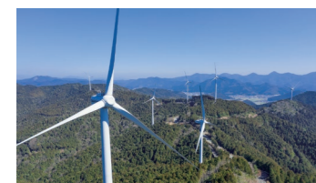
"DREAM Wind Ehime Seijo," capable of producing energy equivalent to that used by approximately 8,000 households (16MW)
