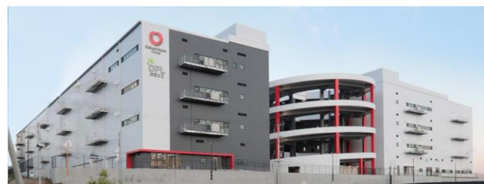
The largest earthquake-resistant multi-tenant logistics facility in Shizuoka Prefecture with a nursery center DPL Shin-Fuji II (completed in April 2020)
