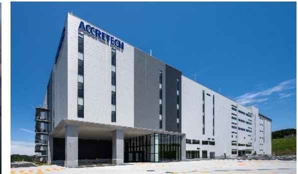
Semiconductor manufacturing equipment manufacturing plant
