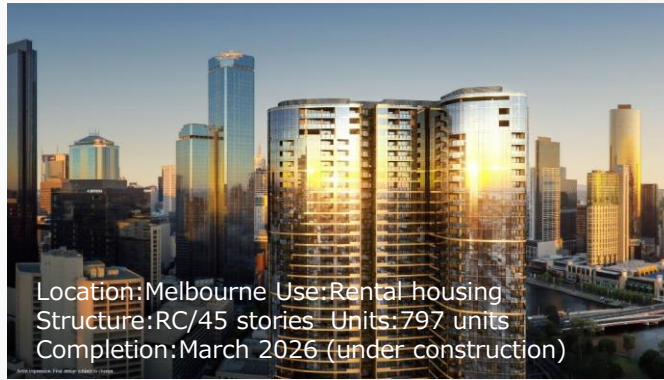
Melbourne Quarter West Project
