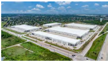
Texas, USA Blue Ridge Commerce Center (5 buildings, Floor area:Approx. 125,000㎡)
