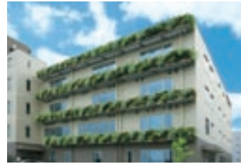
Eco-friendly office: Frame-type "green curtains" fitted to the south side of our Aichi-Kita branch office
