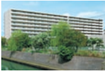
The Premist Inage-Kaigan eco-friendly condominium
