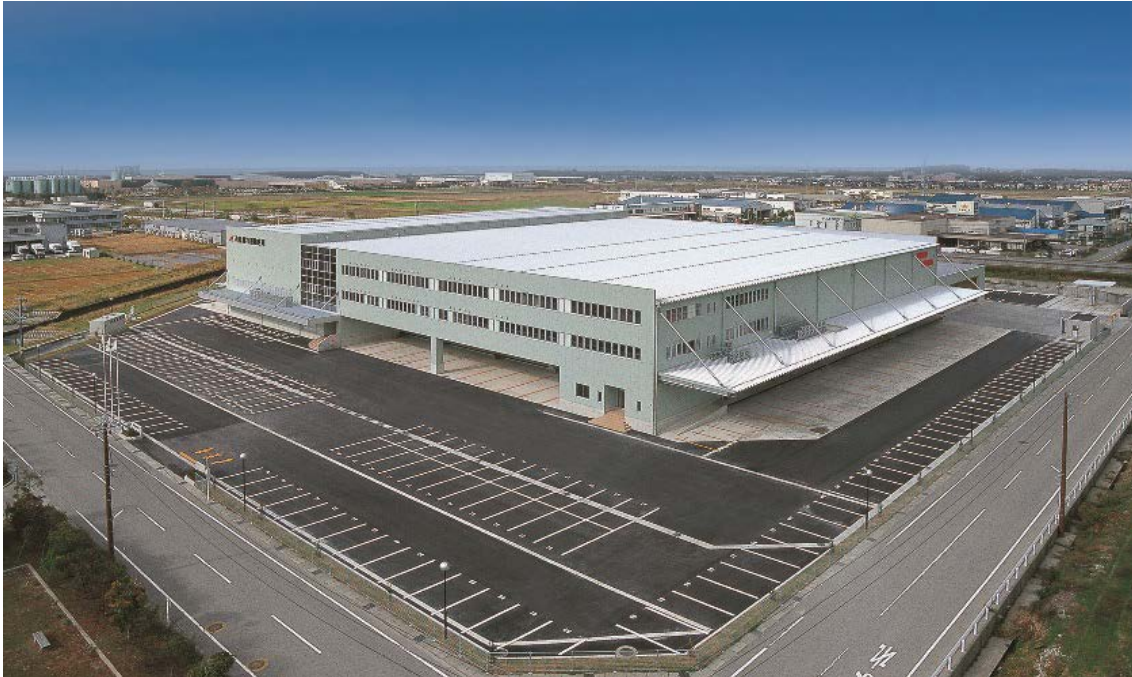
[The four temperature zone joint delivery logistics depot operated by Wakamatsu KONPOU UNYU SOKO]
