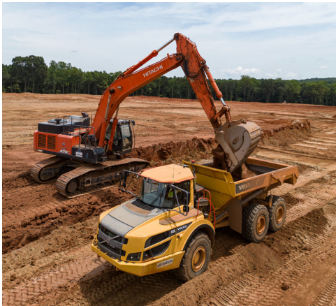
Land preparation work
