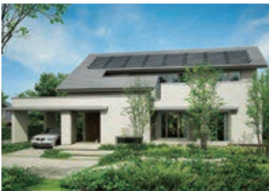
The "SMAxEco ORIGINAL II" smart house, which combines D-HEMS II equipped with storage batteries and air conditioning auto-control technology, a 6.2kWh home-use lithium-ion storage battery, and photovoltaic power generation system
