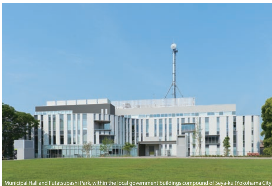
Municipal Hall and Futatsubashi Park, within the local government buildings compound of Seya-ku (Yokohama City)
