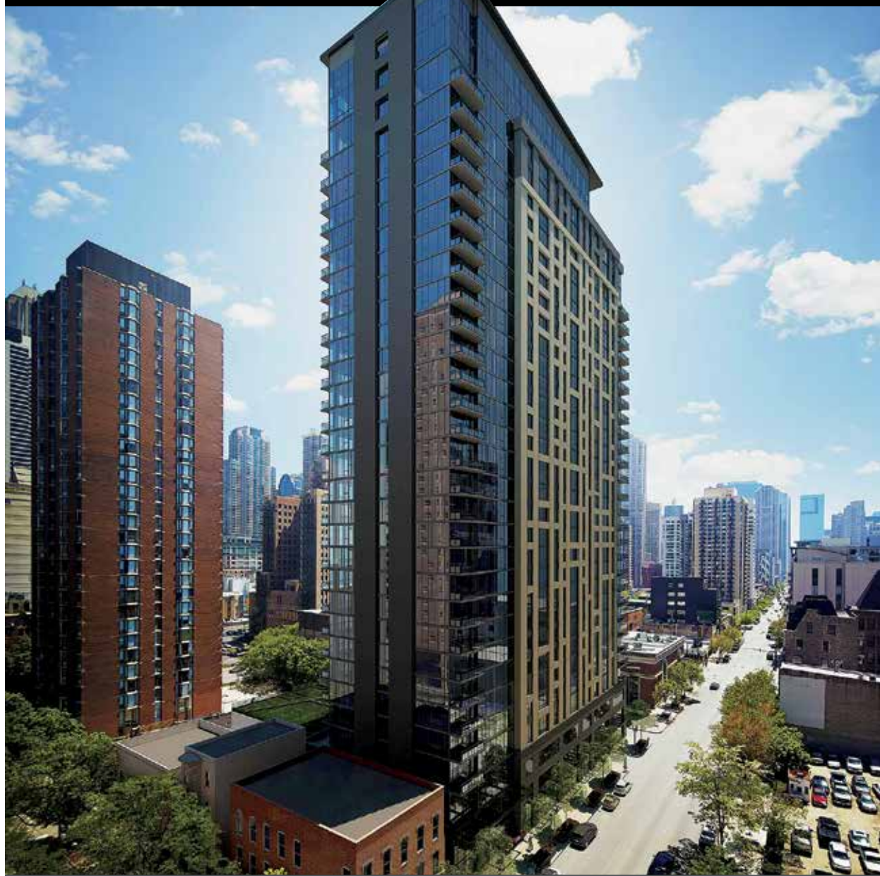
On Chicago's famed Gold Coast, "The Aurélien" is scheduled for completion this spring. The 31-story luxury residence with 368 rental units was developed by partners Daiwa House, Lincoln Property Co. and Ryan Companies U.S., Inc.
