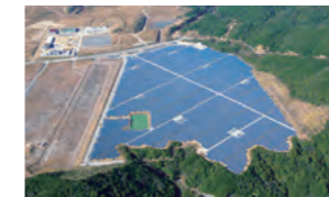
Photovoltaic power generation business
