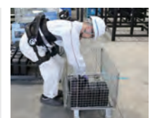
Robot Suit HAL® Application at construction sites
