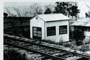
1955 — Pipe House Mr. Ishibashi conceived the idea of a steel-pipe structure, which contributed to resolving the lack of lumber during the postwar reconstruction period.
