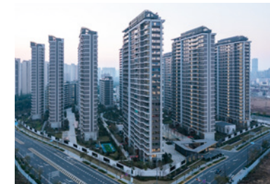
Changzhou Project III
