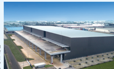
DMLP Phase II Development of a multi-tenant logistics facility in Indonesia
