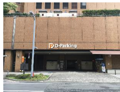
Osaka Marubiru Daiwa House Parking
