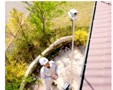
▲ Roof diagnostics "Takamikun"
