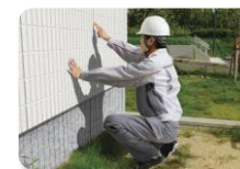
Building inspection/ maintenance extension
