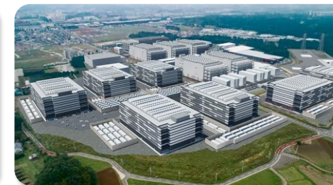
DPDC Inzai (data center)
